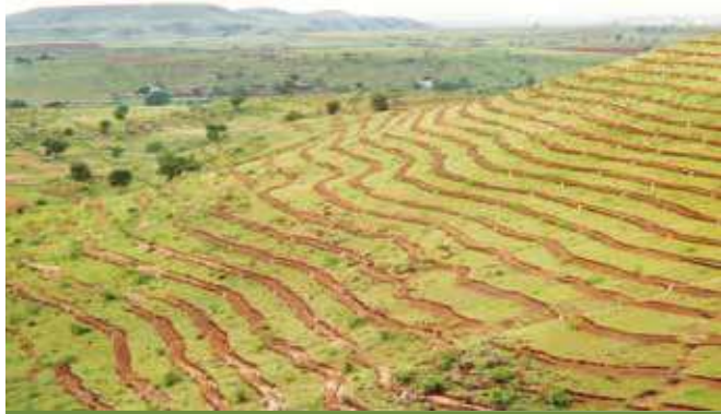
Contour trenching for runoff collection
